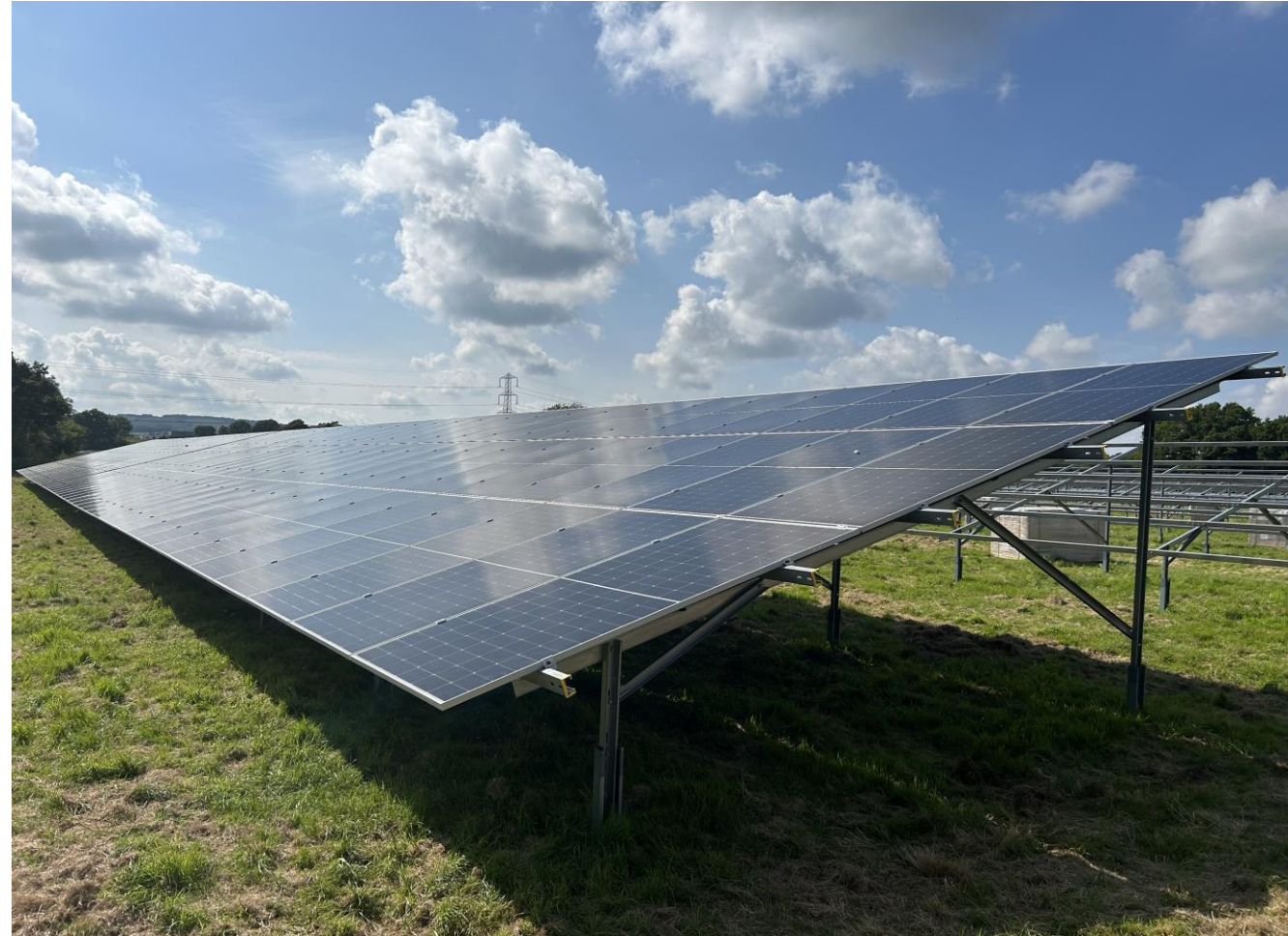
RWE project under construction – Langford (Devon) 15/07/24
